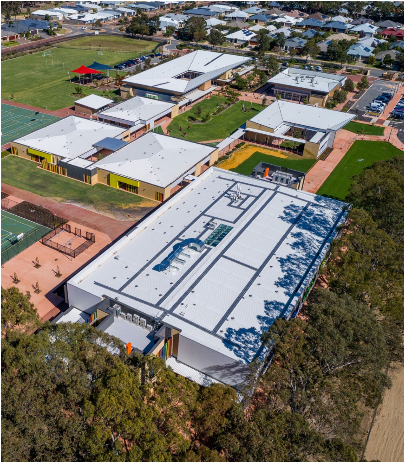
AERIAL VIEW TAKEN FROM THE NORTH-EAST CORNER OF THE STAGE 3 BUILDING, LOOKING WEST TO THE PRIMARY SCHOOL FACILITIES BEYOND
