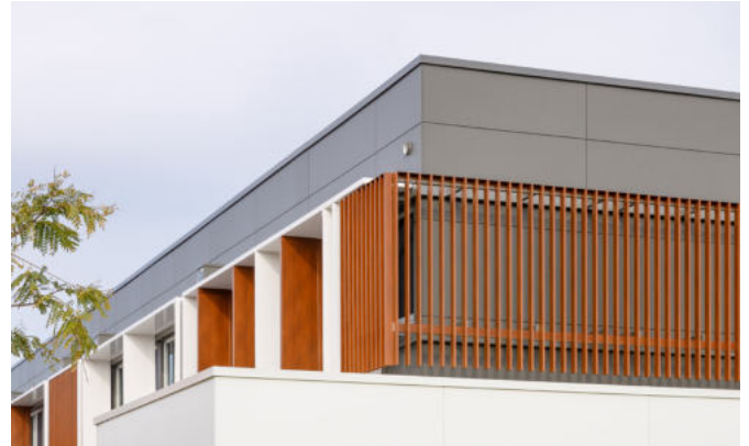
FACADE DETAILS OF THE NORTH-WEST CORNER
