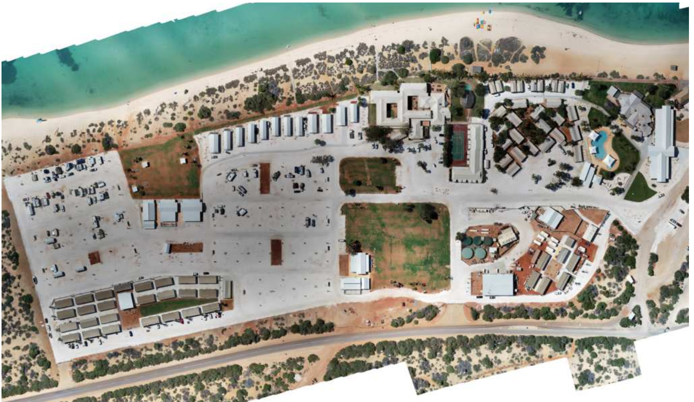
COMPOSITE AERIAL PHOTOGRAPH ON COMPLETION OF THE WORKS
