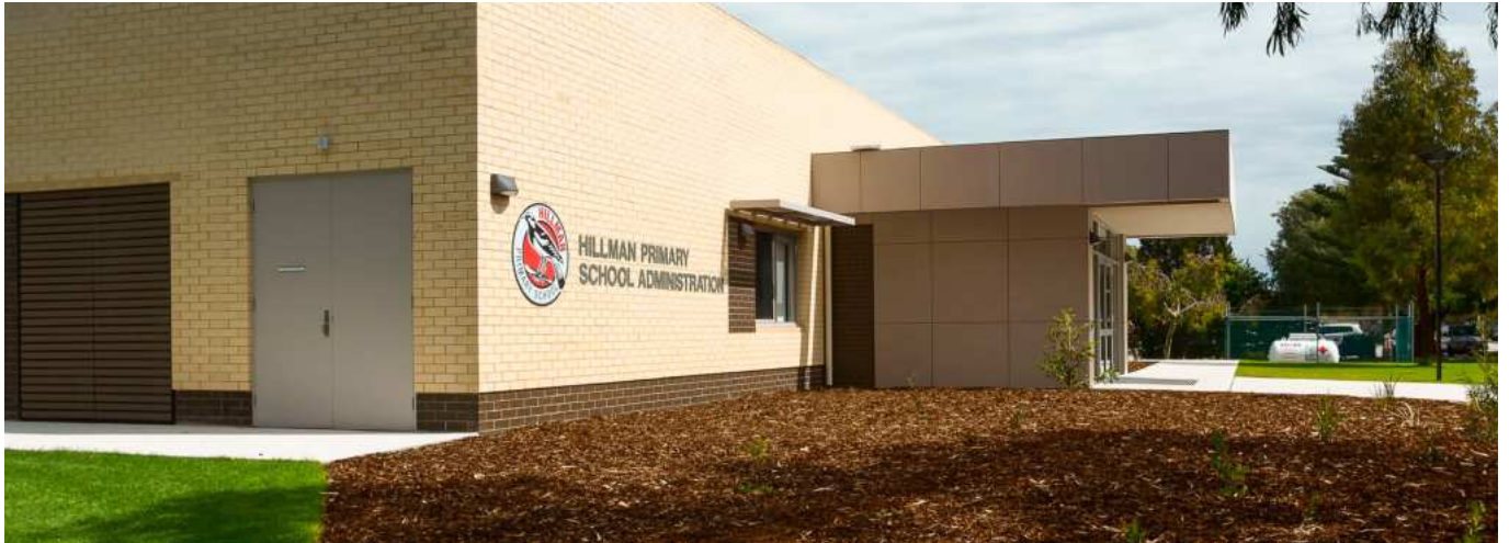
EXTERNAL VIEW FROM NEW CARPARK
