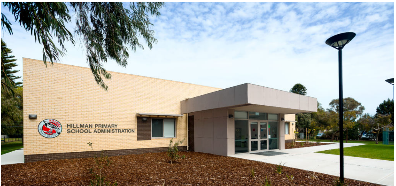
EXTERNAL IMAGE - STREET ELEVATION
