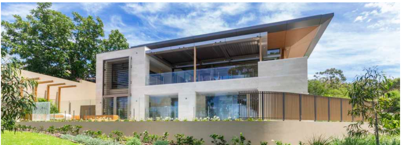
EXTERNAL VIEW OF THE JUXTAPOSED STONE CLAD PLINTH AND SCULPTURAL ROOF LINE
